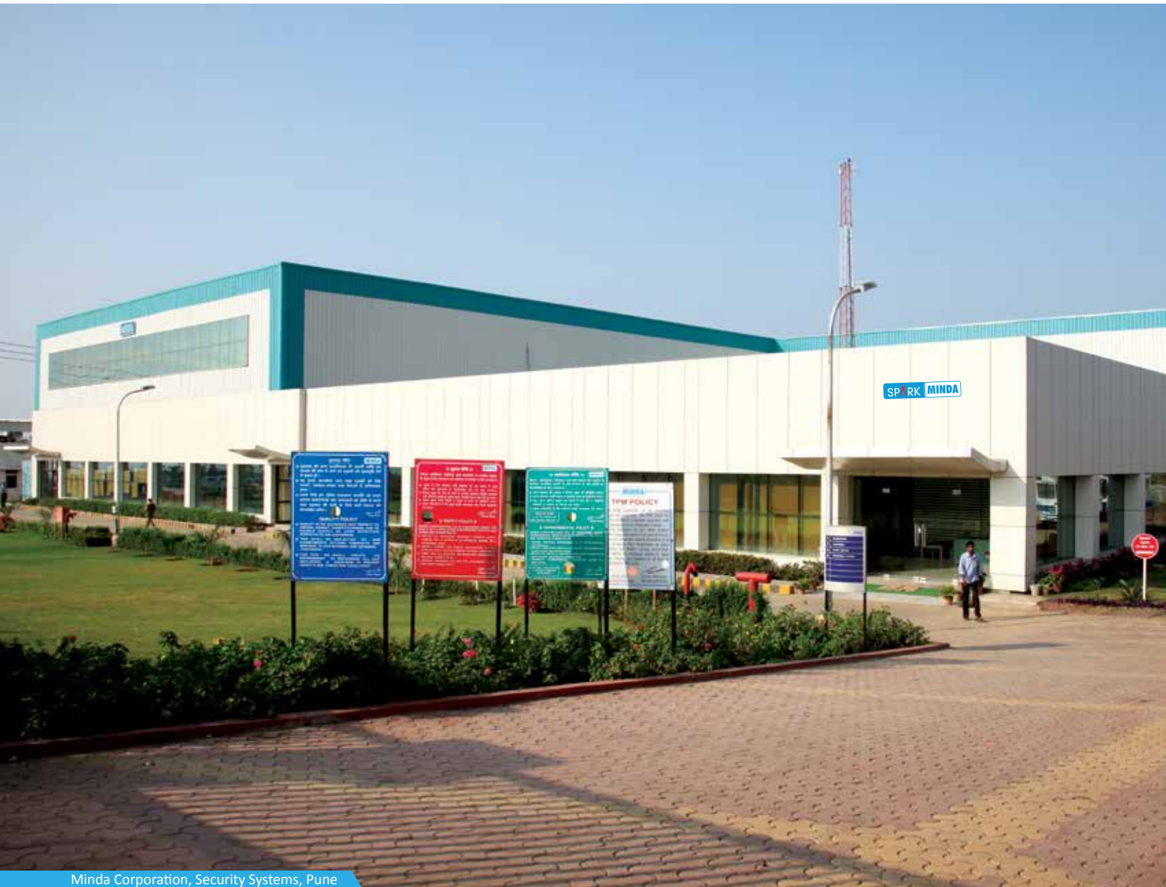
Minda Corporation, Security Systems, Pune
